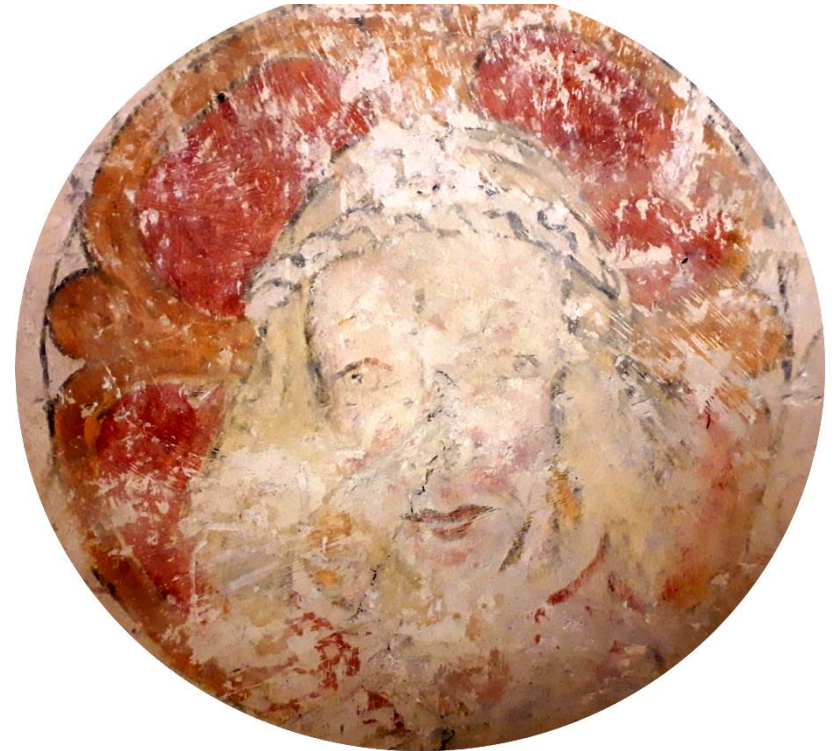
Christ the Crown of Thorns wallpainting in the South Porch
